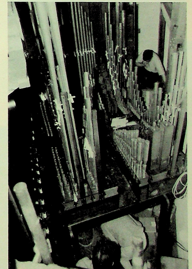
By October, 1969, the Solo Organ Chamber was being filled with chests, reservoirs and pipework and was ready to be wound and wired. The other chamber was also well along but not as complete as this side.
