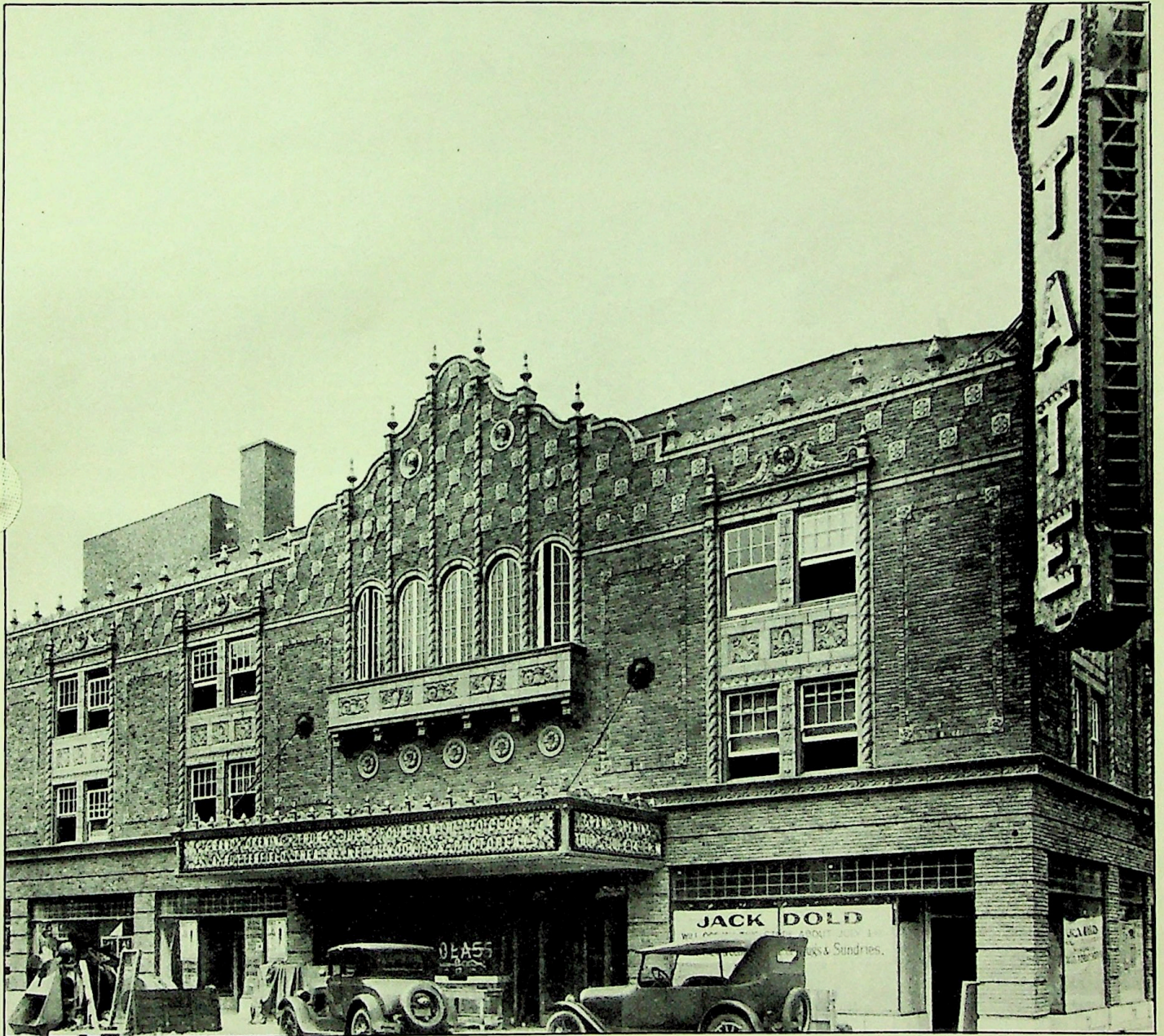
Exterior shot: The Spanish motif was evident on the exterior as well as interior as shown in this circa 1927 photograph. Ornate terr-cotta was used on the building for its entire length along both Burdick and Lovell Streets.
