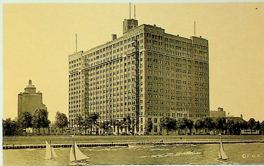
AMERICAN FURNITURE MART BUILDING.
