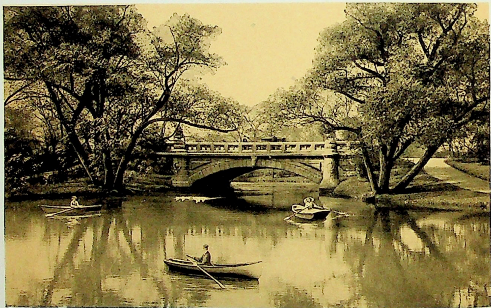
CEMENT BRIDGE, GARFIELD PARK.
