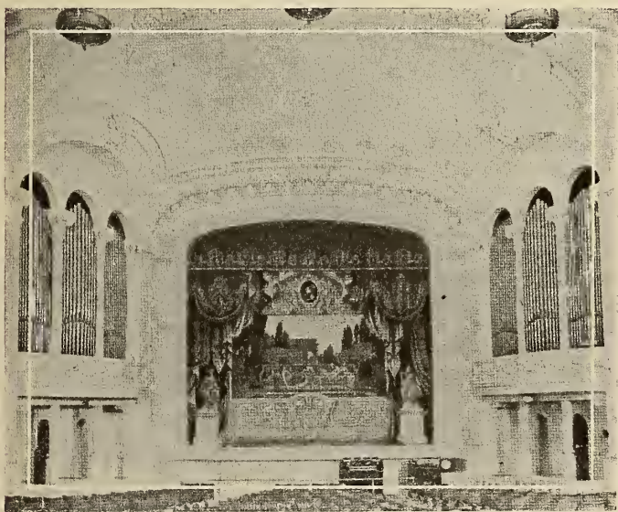
INTERIOR OF A THEATRE SHOWING MEYER ORGAN PIPES INSTALLED
