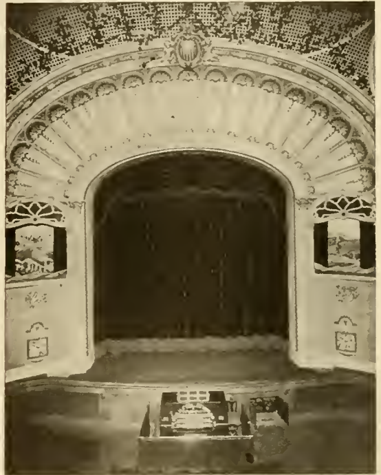
Showing the Effect of Lighting Boxes on Each Side of the Curtain.
